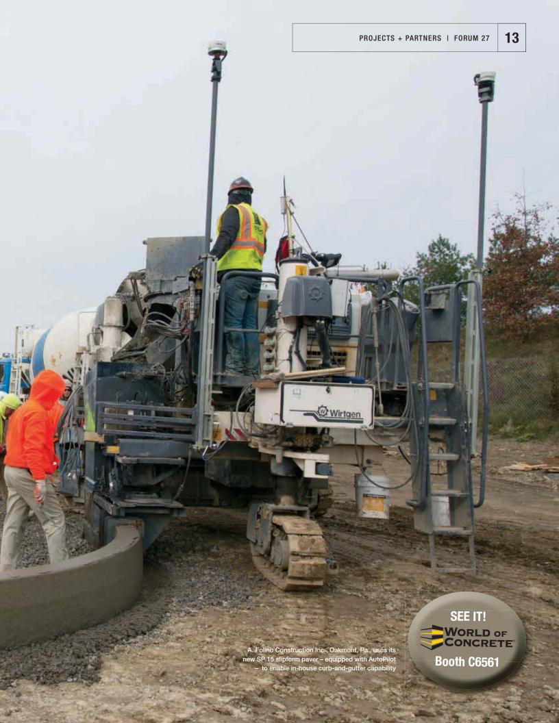
n October 2013, A. Folino Construction Inc., Oakmont, Pa., was using its new SP 15 slipform paver – equipped with AutoPilot – to enable curb-and-gutter capability, and was finding stringless paving to be a huge cost-cutter for curb construction in a competitive arena.
